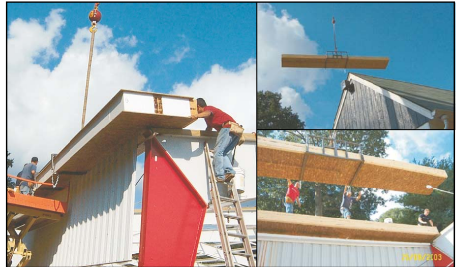
INSTALLATION OF SIP'S
